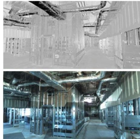
Project buyout scopes for trade partners should specify the right information for FM, formatted the right way. Additionally, the project should think through how it will validate as-built BIMs and data for correctness. Laser Scanning can compare the as-built BIM with installed systems and through tools that check that FM data conforms to the client's data requirements.
