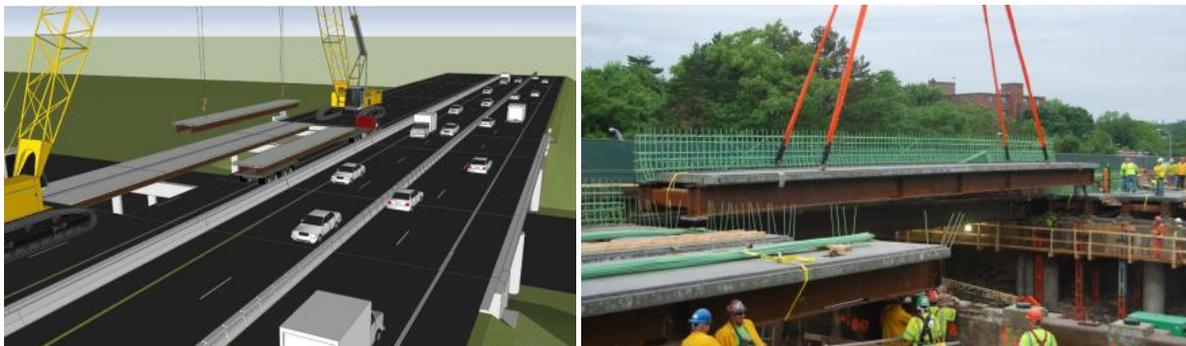
Figures 6 & 7: BIM helped execute the Accelerated Bridge Construction for MassDOT Fast 14 in 2011
