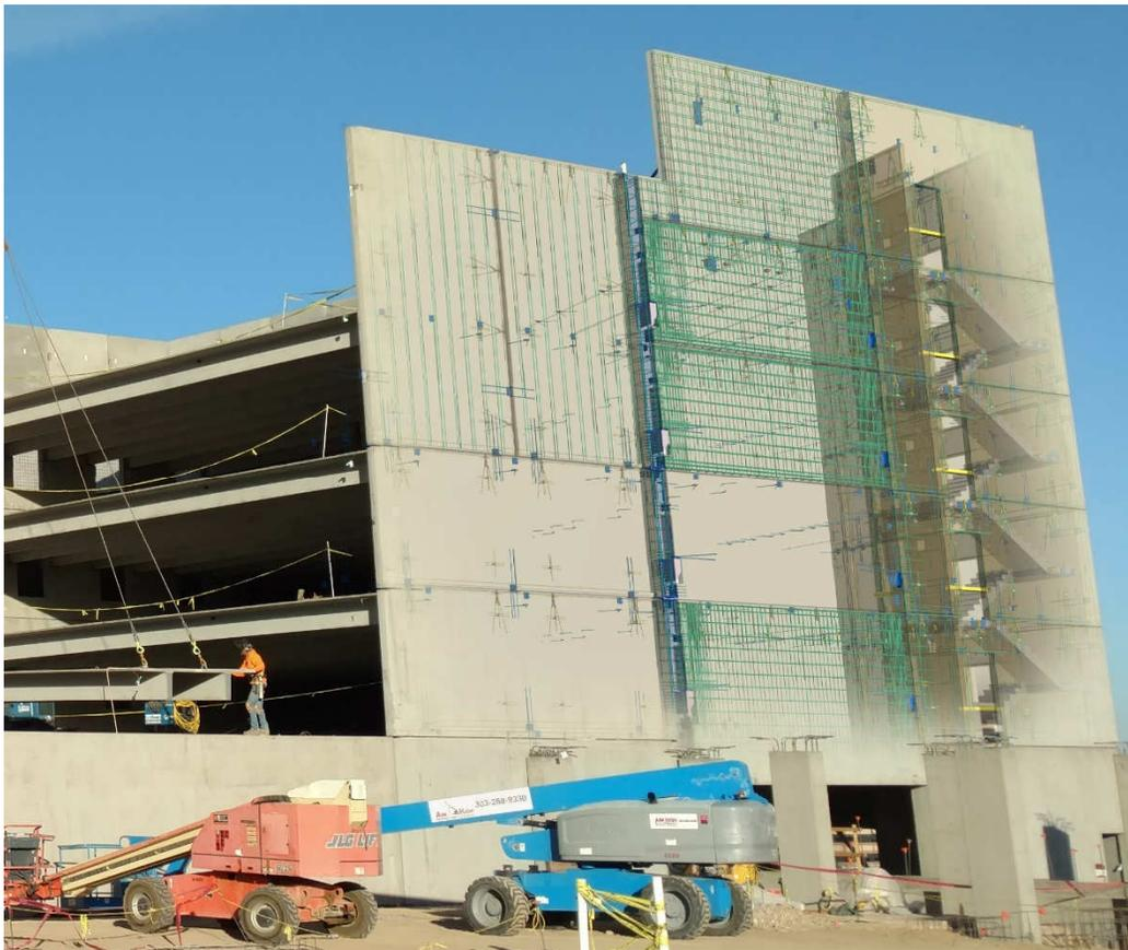
*FIGURE 1: PRECAST PARKING GARAGE, DETAILED USING REVIT, WITH AN OVERLAY OF THE REVIT MODEL*
